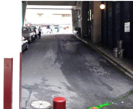
Photograph 6 Blue Anchor Lane West
